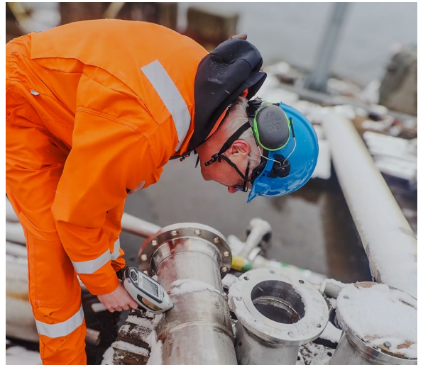
Figure 1. Chemical characterisation of pipe system on-site.
